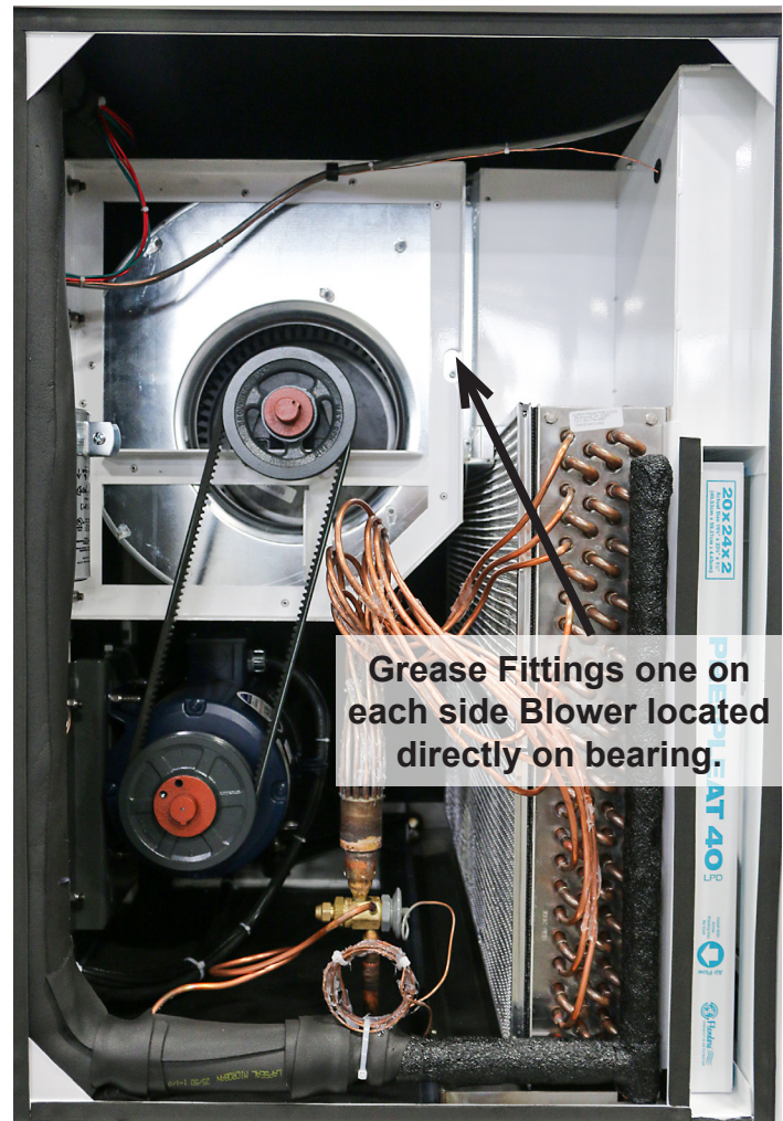
Figure 10 – Evaporator Blower
