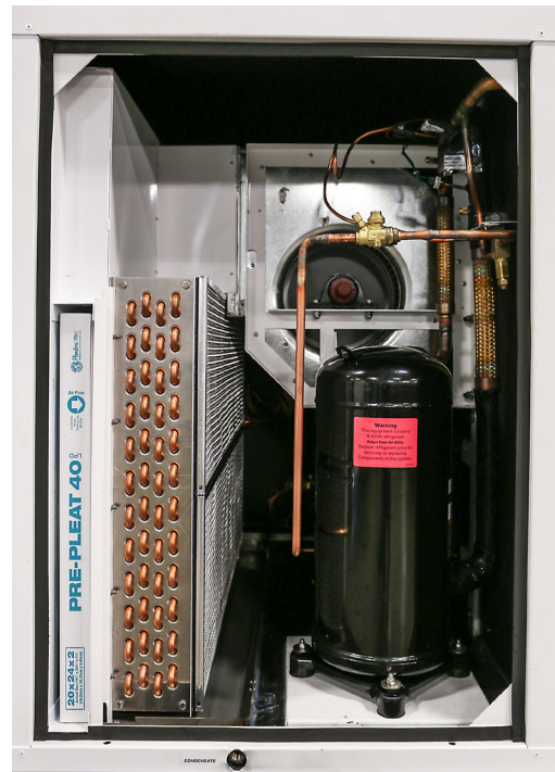
Figure 3 – Compressor Compartment
